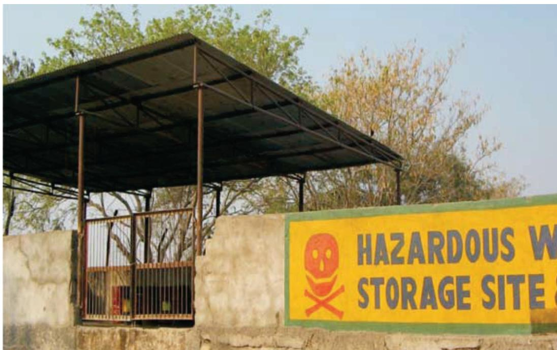
In VC, High performance MOx additive oils are used in critical gear boxes for longer life of oil. Waste oil and Grease is collected in barrels and stored at Hazardous waste storage platform (impervious) with compound wall and tin shed and collected grease is sold to authorized reprocessors and waste oil is burnt in the Kiln. VC had obtained permission/authorization for burning of waste oil in kiln.
